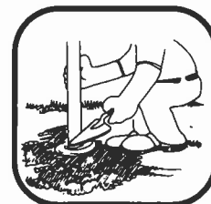
Post aligned and concrete capped.
