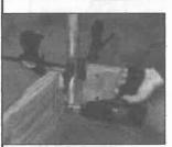
Use the post support as a guide and drill four 1/2" holes through the joists. Insert all four fasteners. Tighten.
