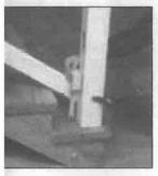
Insert the bottom rall into upper post. Clamp the rail to the lower post at the desired height and angle. Measure the distance from the point where the rail and post meet to the stair tread.
