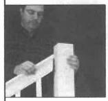
Lift the partially assembled section and insert the top rail into the opening. Push the section down to the deck.
