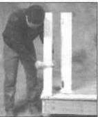
Slide the vinyl post over the brackets. If you intend to use the post trim pieces at the bottom of the post, install them now. Snap them together and slide the assembled trim down the post to the deck.
