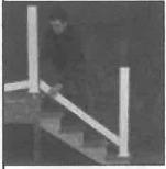
Lift the upper post 3-4" until vou can insert the bottom rail. Then slide the post and rail back down.
