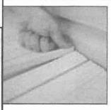
After all the boards have been installed. insert the fill pieces, several at a time. into the channels. Begin by pressing in the leading edge; then slide a block of wood along the length of the fill strips until they are pressed in place.
