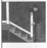
To assemble the rail sections, slide the post over the post support. Insert the bottom rail into the lower post. You may find it easier to lift the lower post, insert the bottom rail, and then lower the post.
