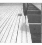
Boards must be fastened every 16". The deck boards are fastened directly to the substructure with #8 x 2" deck screws. Seat the screws in the channels of the plank and do not overtighten the screws.
