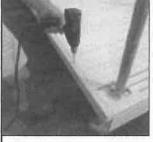
Drill 1/4" holes through the top of the "C" channel. Drill at 1' increments (in the center of every other plank). Press the end-cover fasteners through the holes into the deck.
