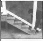
Lay the bottom rail between the posts. with the end holes clear of the posts and equally spaced. Align the rail with the top of the rail on each post. Measure the rail.
