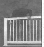
Pull up on the first few balusters and insert them into the top rail holes. Push down on the top rail and position it next to the opening in the post. The rail may not easily push into the post opening until you have inserted several balusters.
