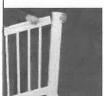
Once all balusters are inserted, lift the partially assembled section and insert the top rail into the post opening. Push the completed section down to the deck.
