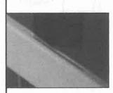
Use care when installing glass balusters. Insert glass balusters the same way. To fit properly, the angle cut on the glass baluster needs to be installed in the same direction as the stair angle.
