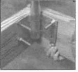
Recheck level; if the joists are not plumb, use a washer as a shim to level the post support. Install deck boards.
