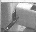
Pre-drill 9/64" hole for rail attachment screw.
