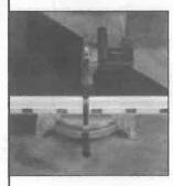
Cut the bottom rail, keeping the aluminum approximately 1/4° shorter than the vinyl. Use the bottom rail as a guide to cut the top rail.
