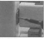
Drill pilot hole with a 9/64" drill bit for bracket attachment screw.
