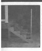
Begin the stair section by installing the stair post support and E-Z Set brackets. Do not cut the support posts vet.
