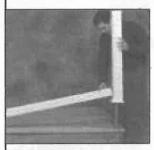
Lift the next post and insert the rail into opening. Push the post and rail down to the deck.
